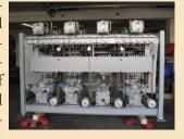
and waste-cooling as well as the chilled water units. Imtech Marine implemented a number of notable innovations for the German Navy. In the fresh air supply of the modular air filtration unit for example, Imtech implemented a humidity control with a compulsory emptying of chillers and heaters in case of freeze alarm, in order to protect the system.
