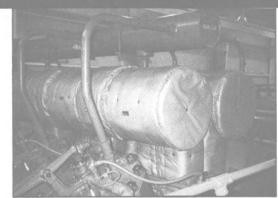
INSULTECH Thermal Blankets were used on a D-R TCV-10 Sectional Manifold. Blankets were custom fit via CAD.
