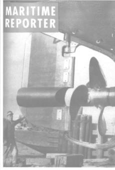
Pictured on the cover of the January 1, 1953 edition of Maritime Reporter is a close up of the rudder and propeller assembly of the Dalzellera, the first harbor tug in the U.S. to be equipped with the new controllable pitch propeller. The 100-ft. pioneering tug was operated in New York harbor by the Dalzell Towing Company.
