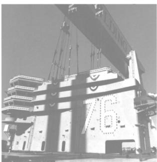
Ronald Reagan (CVN-76) features a completely redesigned pilothouse — the first major redesign, and the first ever designed using 3-D product modeling. The opening at the aft end brings the on-deck weapons elevator under cover, allowing for weapons handling during flight operations.
