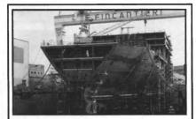
FROM TWO TO ONE: Disney's two cruise ships were each built in two sections at two different shipyards — Fincantieri's Ancona yard and Fincantieri's Marghera yard - in order to complete the vessels as quickly as
