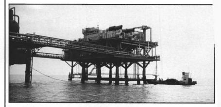
Pictured is an offshore platform with two Heatec waste heat recovery units.
