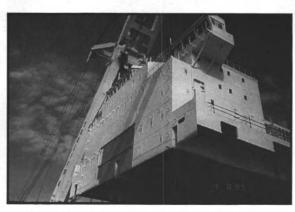
The Taklift 4 is shown lifting the accommodation block for the Stolt Innovation into place.
