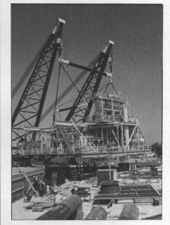
Using a unique three-bar spreader system the derrick barges Cappy Bisso and Lili Bisso, of Bisso Marine Company, load out Shell Oil's 960-ton production module for the BUD platform M.P. 252 "A.
