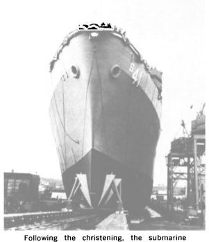
tender McKee (AS-41) slides down Lockheed Shipbuilding and Construction Company's shipway on Harbor Island and enters the West Waterway of the Duwamish.
