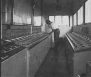
Control of pumps and flooding for all 40 ballast compartments through banks of buttons and indicators is centered here in the control house atop the west wingwall.
